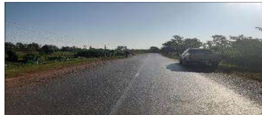
Plate 0-4: Houay Saiphai Bridge (Km 73+730)
