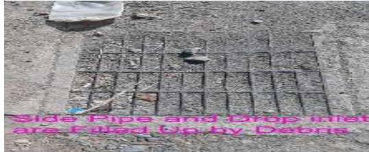
Plate 0-10: Side Pipe and Drop Inlet are Filled Up by Debris
