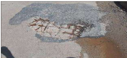
Plate 0-15: Nam Don Bridge with Surface Deteriorated
