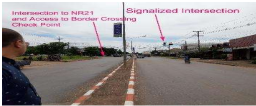
Plate 0-9: Urban Road in Paksan Township
