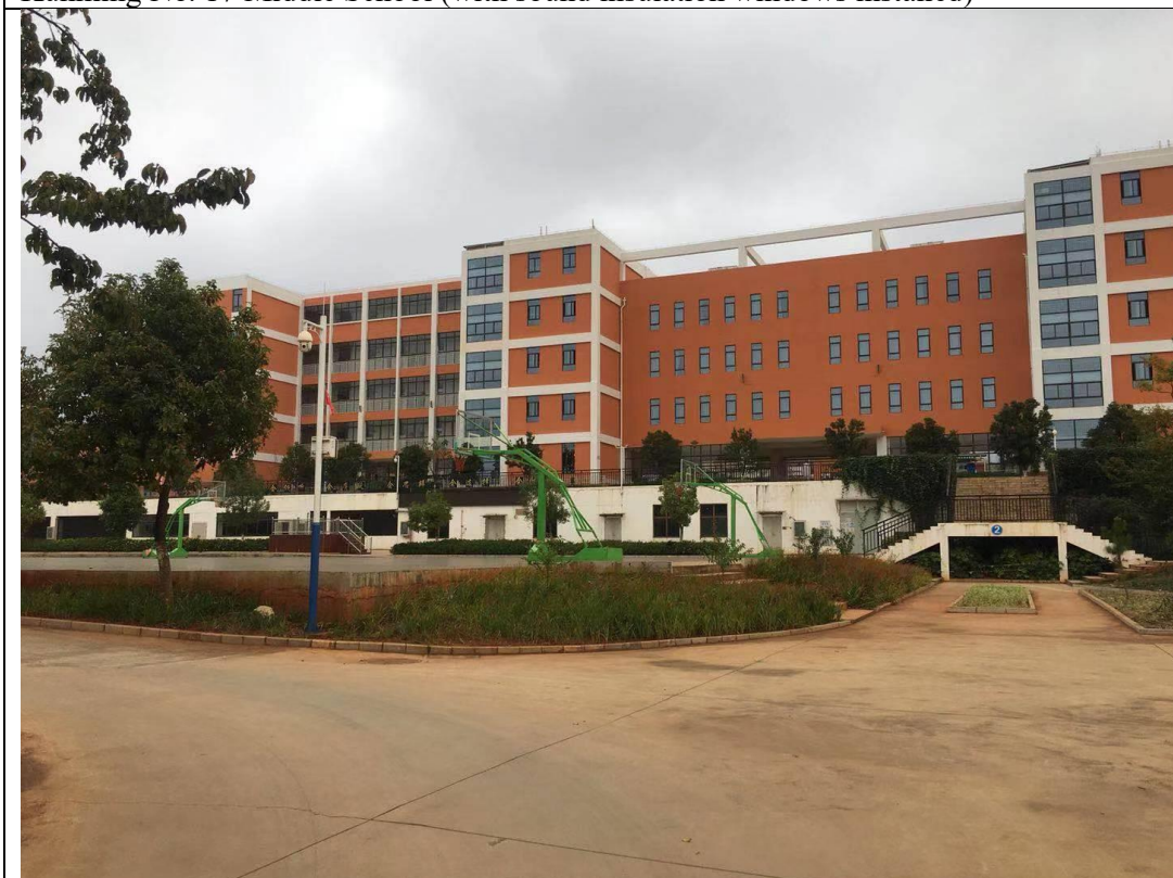
Kunming Airport No.1 Primary School (with sound insulation windows installed)
