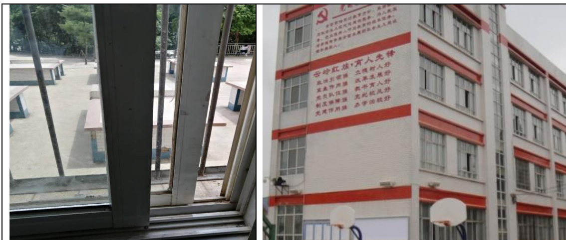
Shagou Primary School (with sound insulation windows installed)
