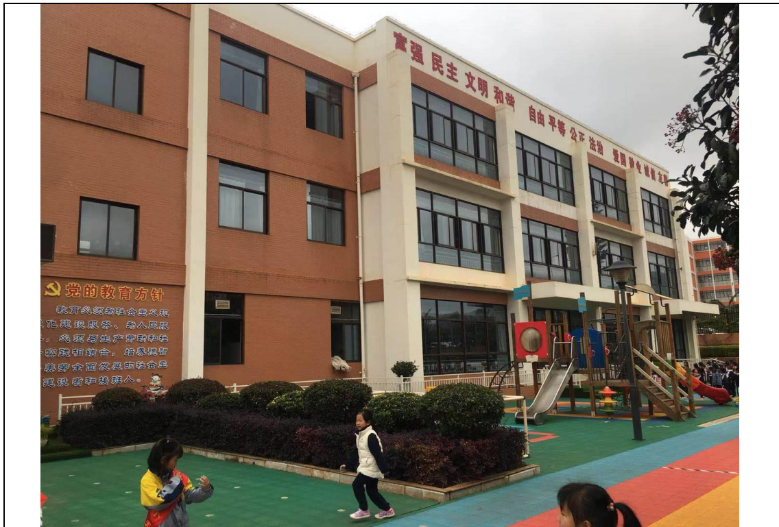
Kunming Airport Economic Zone No.1 Kindergarten (with sound insulation windows installed)
