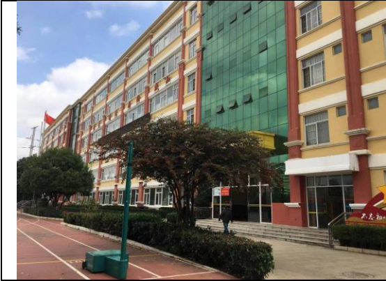
Airport Experimental School of Kunming No.3 Middle School
