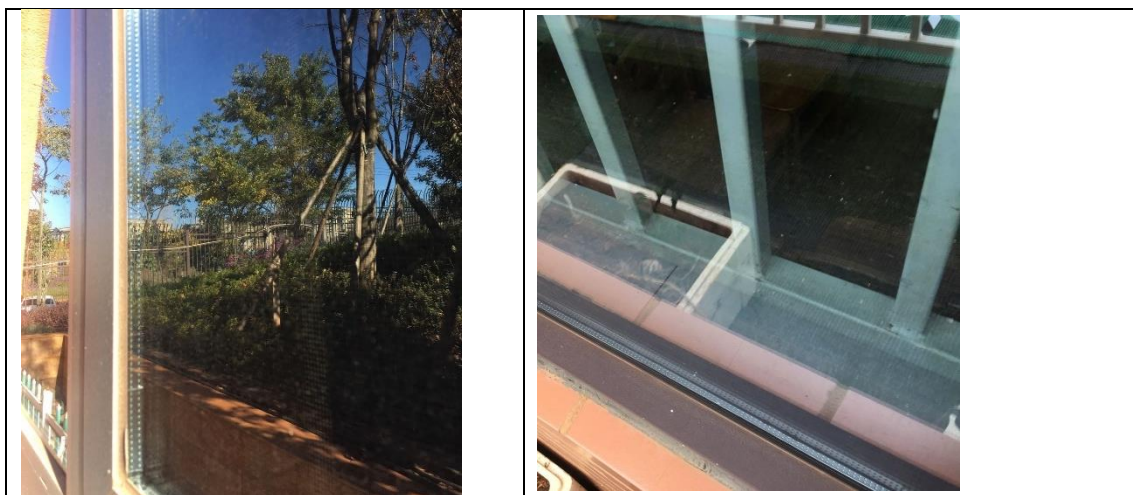
Example of hollow double-layer casement sound insulation window
