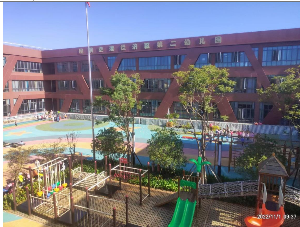
Kunming Airport Economic Zone No.2 Kindergarten (with sound insulation windows installed)
