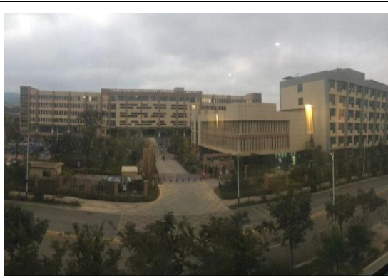
Kunming No. 17 Middle School (sound insulation measures installed)
