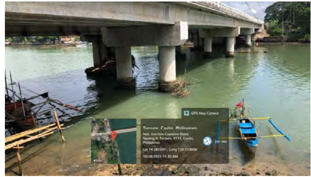
K0056+157 (Maragondon Bridge)
