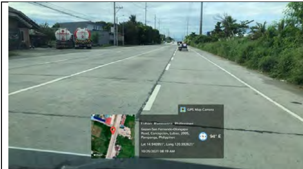
K0086+900 (Santa Cruz Bridge)
