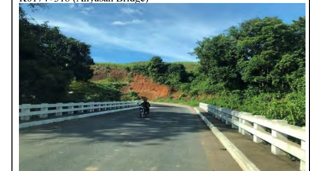
K0169+254 (Binuangan Bridge)
