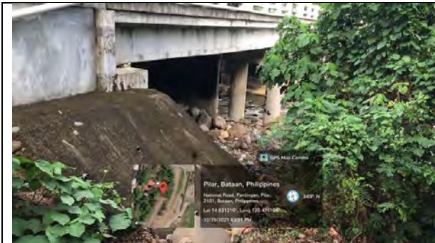
K0137+013 (Pantingan Bridge)
