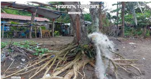
Exposed roots due to high tidal waves during typhoons Tisoy and Rolly occurred in 2019 and 2020, respectively along Brgy. Timalaya Concepcion, Naic, Cavite
