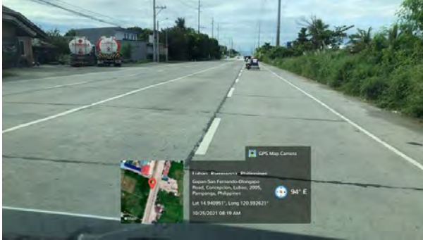
K0086+900 (Santa Cruz Bridge)
