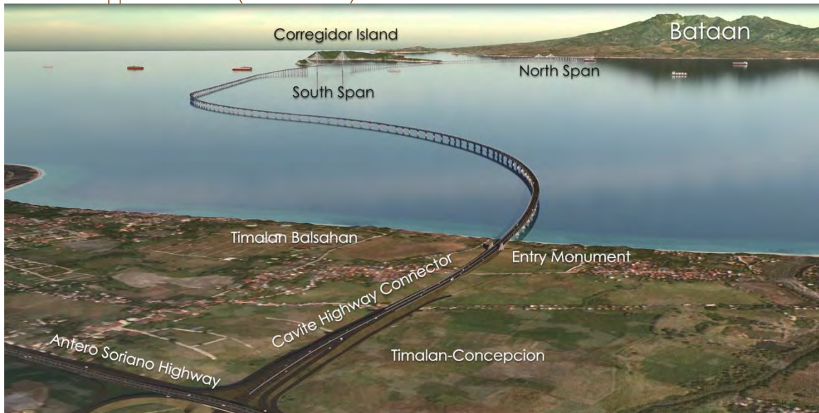
Exhibit 3: Approach Road (Cavite Side)
