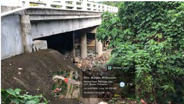
K0137+013 (Pantingan Bridge)
