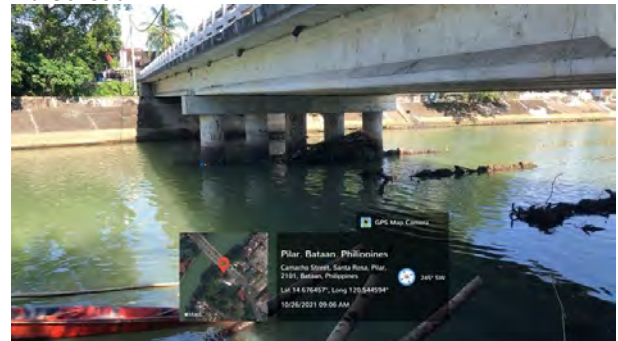
K0132+450 (Orion Bridge)
