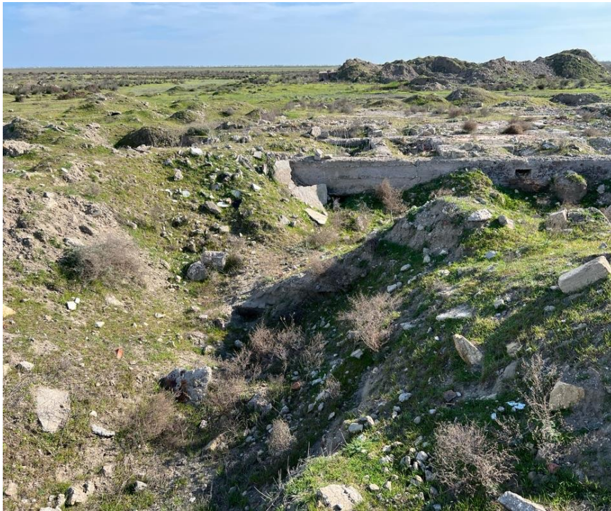
Signs of recent historical dirt moving by heavy machinery are abundant at the site, with many artificial ditches and berms present.
