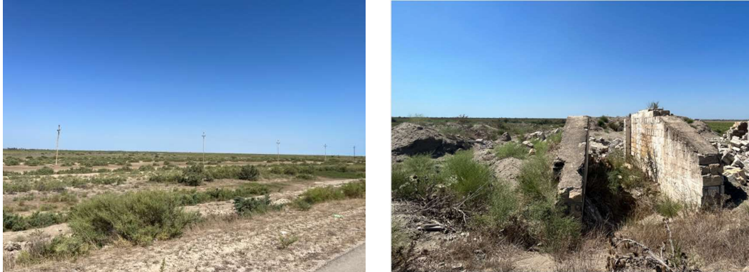
Figure 2-5 Site Features: Existing OHTL (left) and Military Building Ruins (right)
