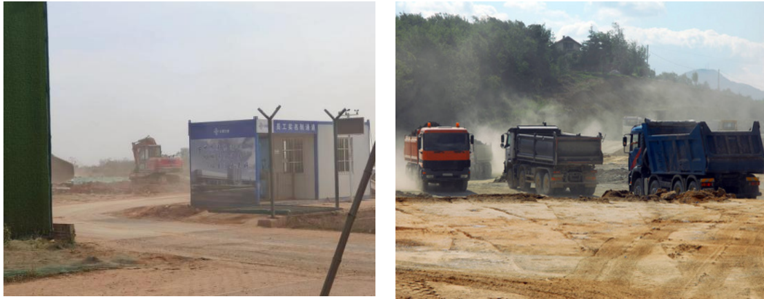
Figure 8.5-7 Project Construction Site
