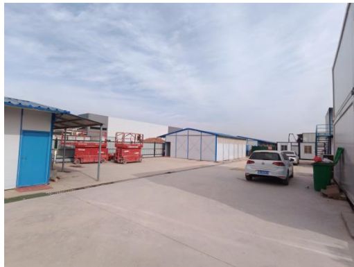
Construction Camp of the Advanced Project Activities
