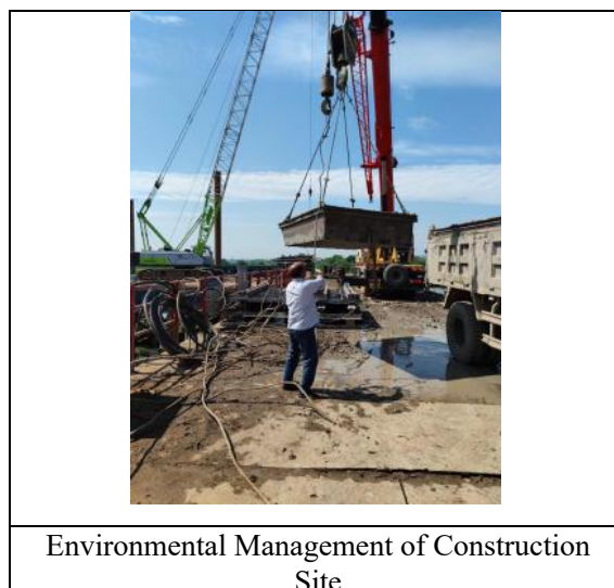
Figure 1.5-8 Site Situation and Supporting Photos of Environmental Management
