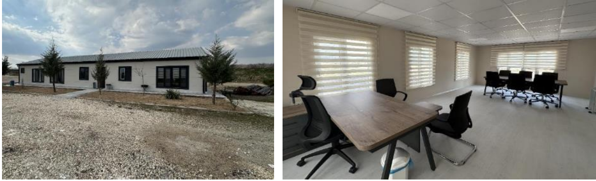
Figure 89. Tohma Camp Site
